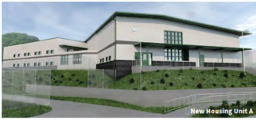
New Housing Unit A
