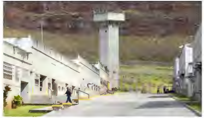
Halawa Correctional Facility ("Prison") (Credit: Honolulu Star Advertiser)
