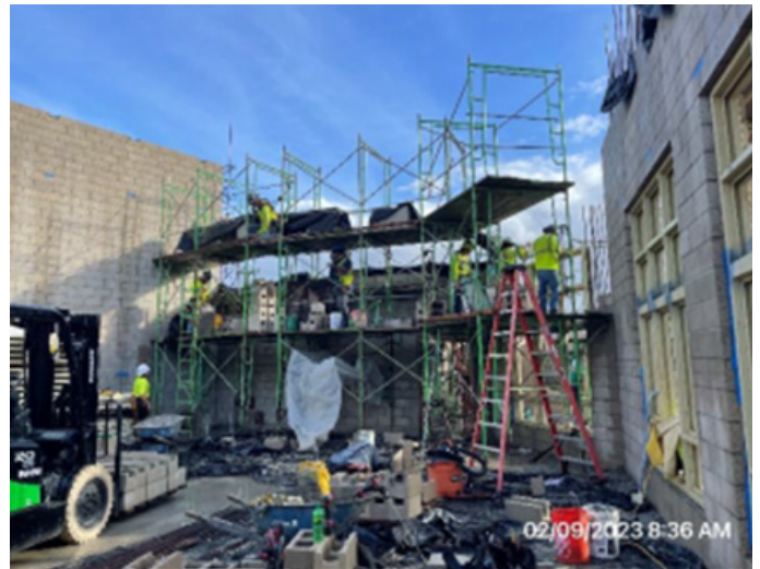
CMU installation in progress at the dayroom's south wall (Credit: Rider Levett Bucknall)
