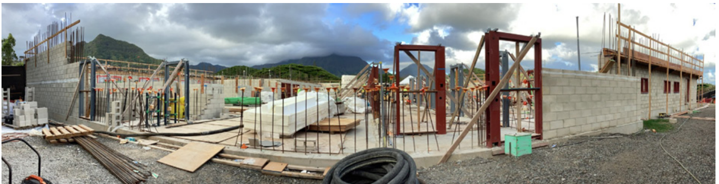
Construction Progress Photos, September 2022 (Rider Levett Bucknall)
