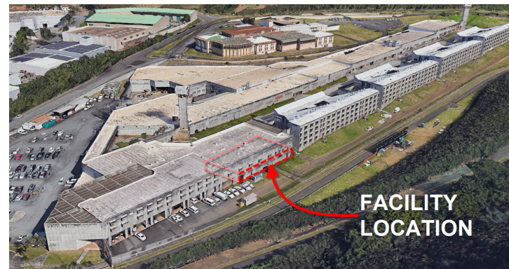
Location of New Consolidated Health Care Unit at HCF. Credit: Mitsunaga/Arrington Watkins Team
