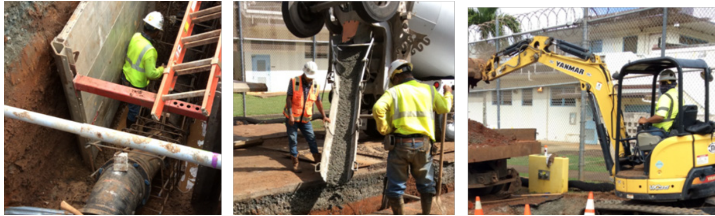
WCCC construction progress photos (December 2021/January 2022)
