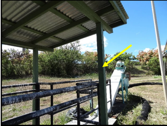
HM ID: 31 Pre-Treatment Plant
