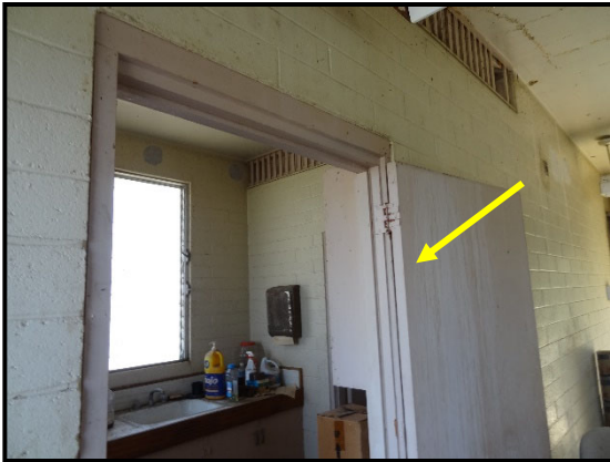
HM ID: 17 Pre-Treatment Plant
