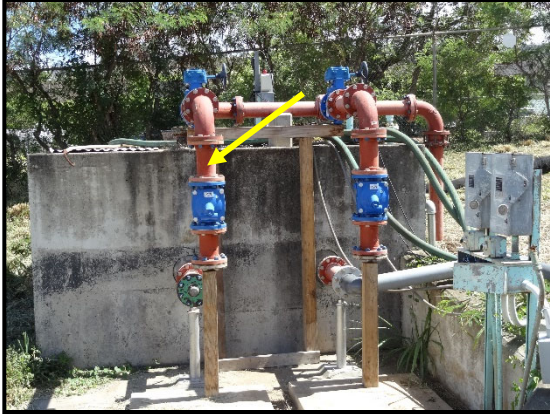
HM ID: 34 Pre-Treatment Plant
