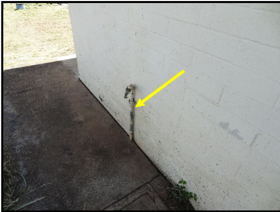
HM ID: 29 Pre-Treatment Plant
