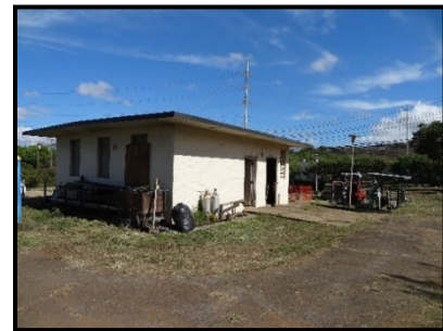
Pretreatment Plant and Shed
