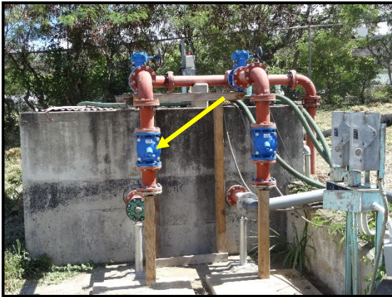
HM ID: 35 Pre-Treatment Plant
