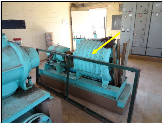
HM ID: 18 Pre-Treatment Plant
