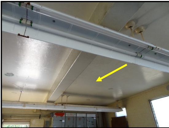
HM ID: 14 Pre-Treatment Plant
