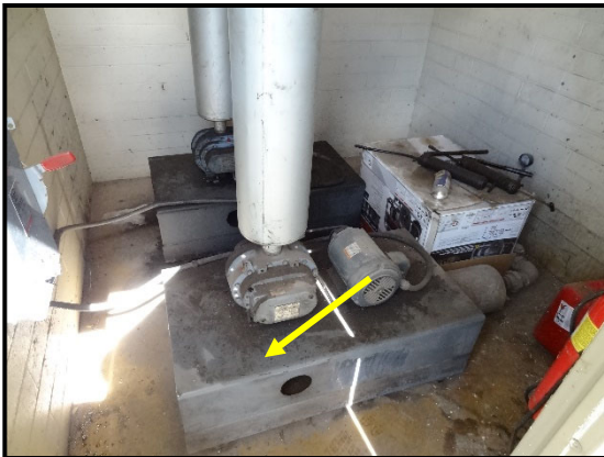
HM ID: 36 Pre-Treatment Plant
