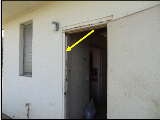
HM ID: 28 Pre-Treatment Plant
