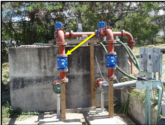
HM ID: 30 Pre-Treatment Plant
