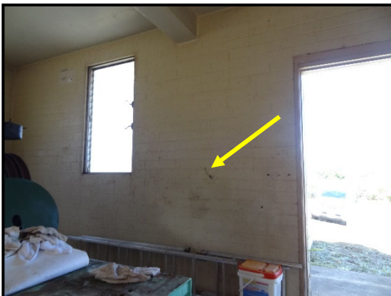
HM ID: 15 Pre-Treatment Plant
