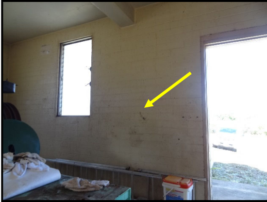
HM ID: 16 Pre-Treatment Plant
