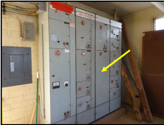
HM ID: 20 Pre-Treatment Plant
