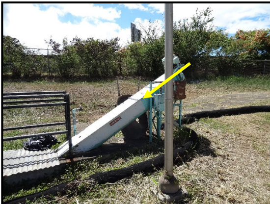
HM ID: 33 Pre-Treatment Plant
