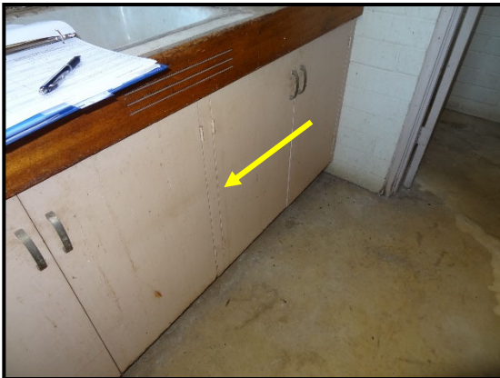
HM ID: 21 Pre-Treatment Plant
