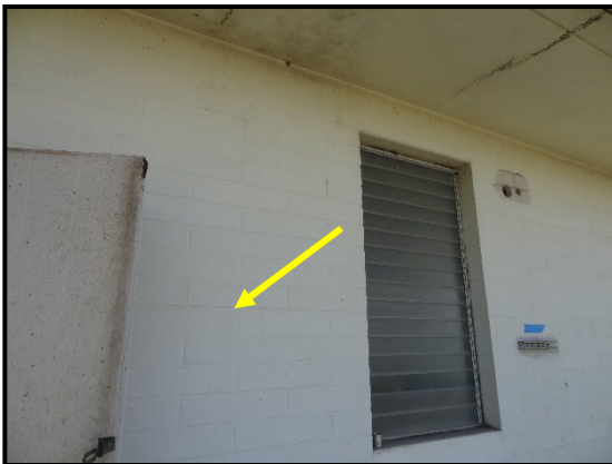
HM ID: 27 Pre-Treatment Plant
