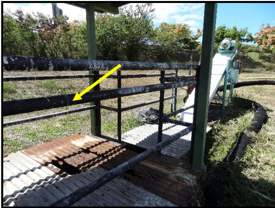
HM ID: 32 Pre-Treatment Plant
