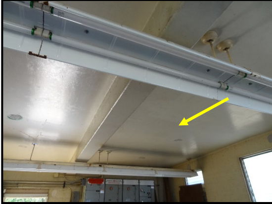
HM ID: 13 Pre-Treatment Plant
