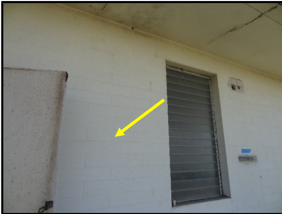
HM ID: 26 Pre-Treatment Plant
