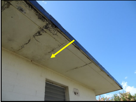
HM ID: 25 Pre-Treatment Plant
