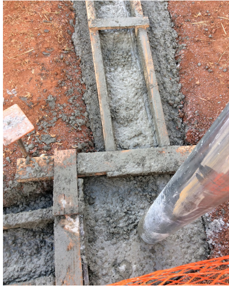
Concrete pour for temporary security fence grade beams underway.
