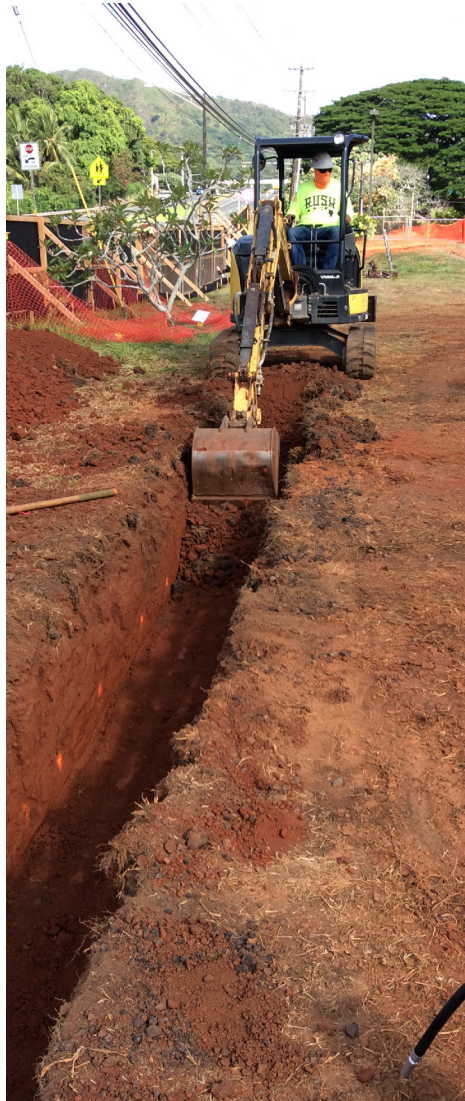
Excavation for temporary water line install near Kalaniana'ole Highway.
