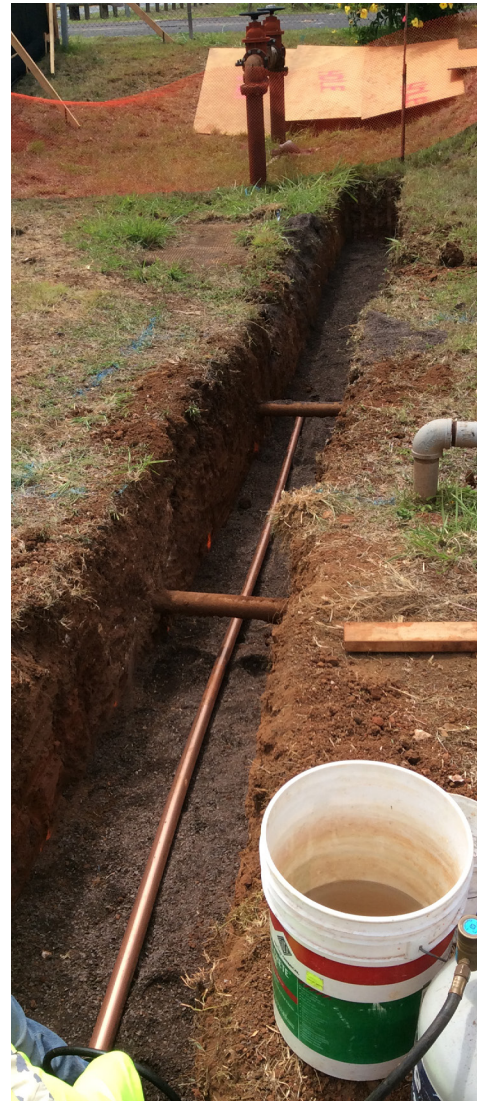
Two-inch copper pipe installed for temporary water line for administration trailers.
