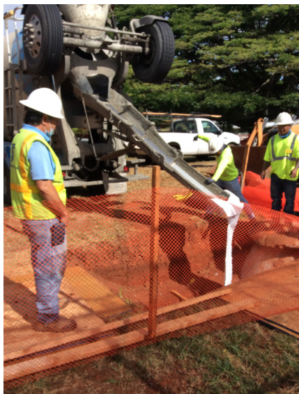
Concrete pour for temporary sewer line connection to manhole
