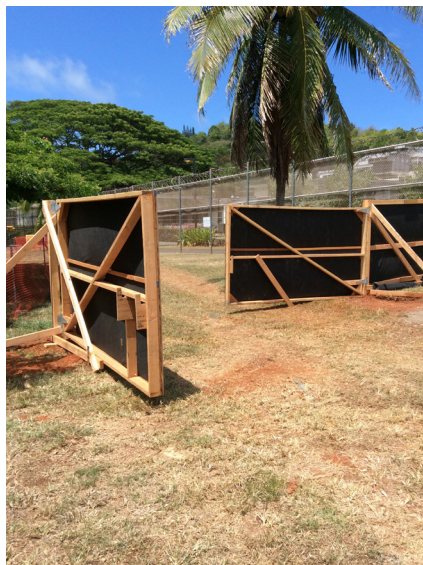
Gates installed for temporary dust fence for heavy equipment access.
