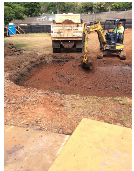
Excavation underway near main entrance for new sediment basin.
