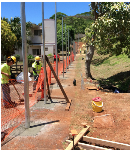
Temporary security fences posts installed.
