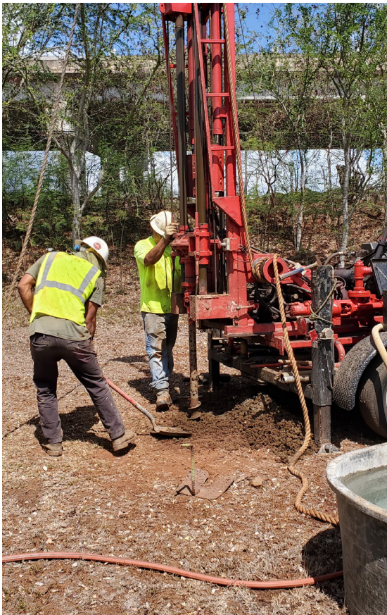
OCCC team members conducting soil borings and hazmat sampling at site of new AQS.
