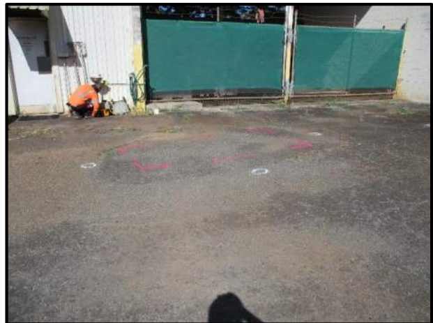
Former UST Area at the Maintenance Shop where TPH-DRO exceeded the EALs.
