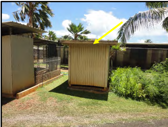
HM ID: 112 Electrical Shed Floor 1
