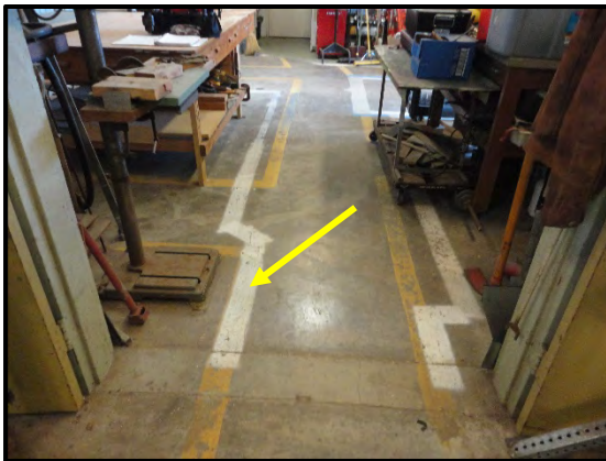
HM ID: 220 Maintenance Shop Floor 1 Warehouse White paint on concrete floor.
