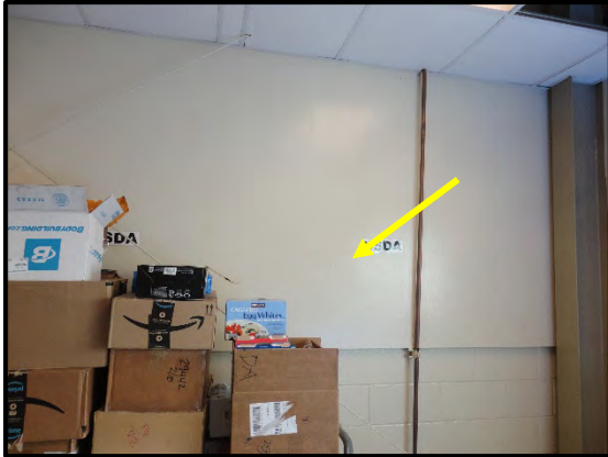
HM ID: 231 Maintenance Shop Floor 1
