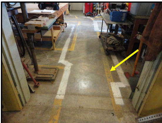
HM ID: 221 Maintenance Shop Floor 1 Warehouse Yellow paint on concrete floor.
