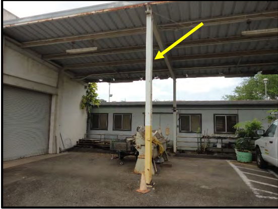
HM ID: 200 Maintenance Shop Floor 1 Exterior White paint on metal conduit.
