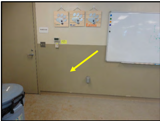
HM ID: 232 Maintenance Shop Floor 1
