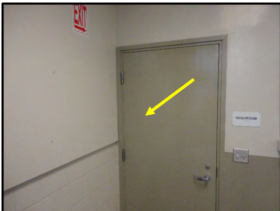
HM ID: 233 Maintenance Shop Floor 1
