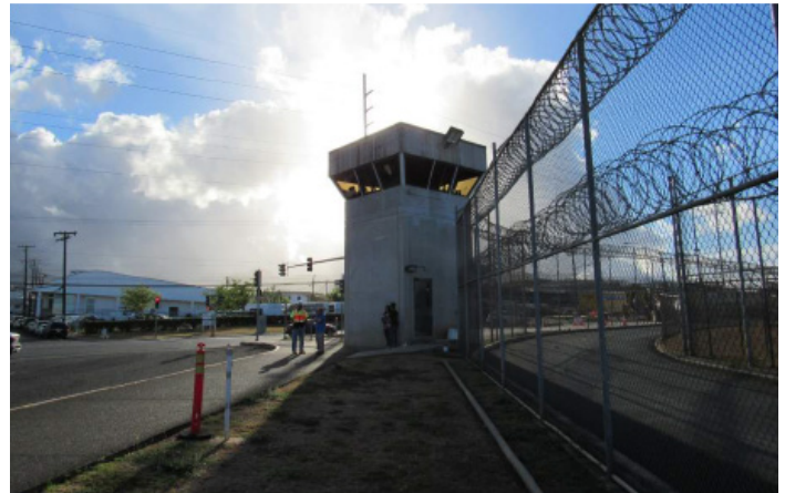
Guard tower at existing Oahu Community Correctional Center
