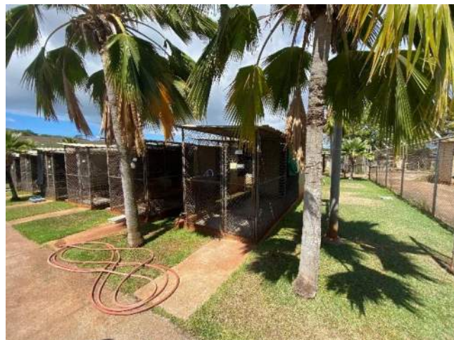
Photo-41: Water Hose Connection
