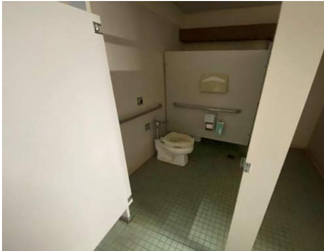
Photo-31: ADA Toilet Stall
