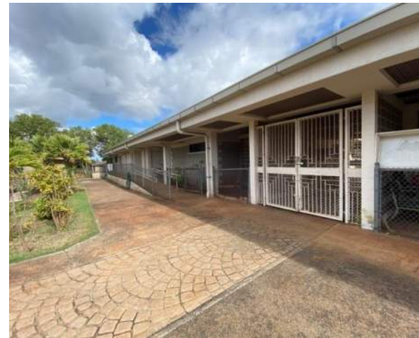
Photo-5: Secured QAC Gate and Public Vestibule
