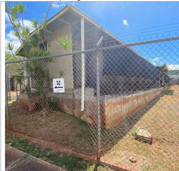
Photo-53: Trench Drain along Length of Cattery
