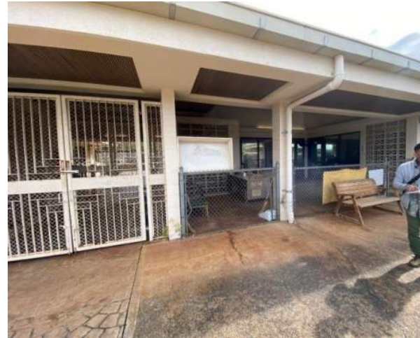
Photo-3: QAC Gate & Public Vestibule
