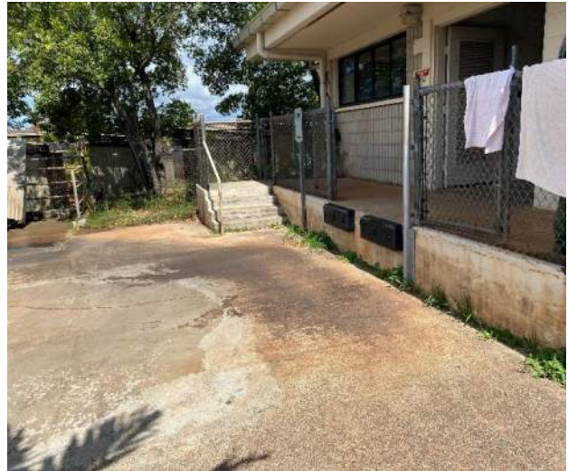
Photo-25: QAC Loading Dock
