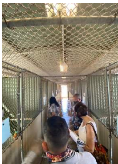
Photo-56: Double Loaded Corridor
