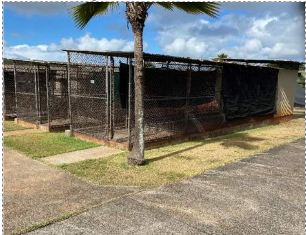
Photo-42: Typ. Kennels with Trench Drains along Length
