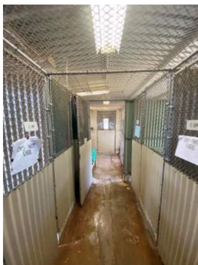
Photo-55: Double Loaded Corridor
