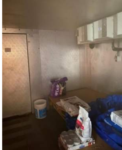
Photo-27: Freezer Room
