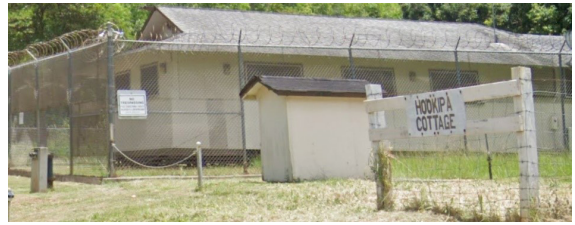
Existing Ho'okipa Makai Cottage
