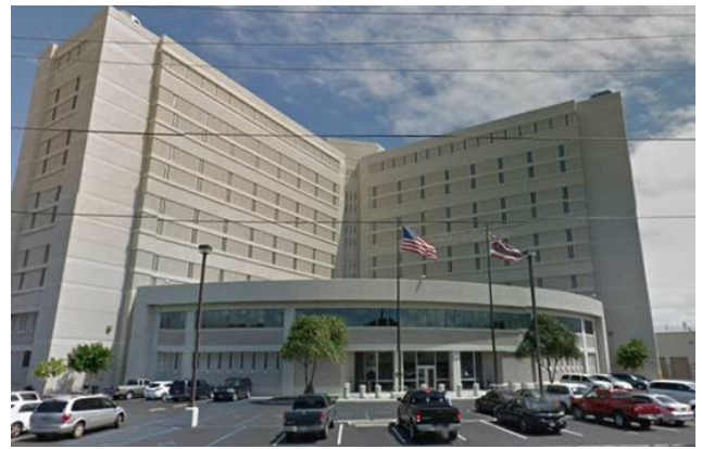
Federal Detention Center in Honolulu (i.e., jail).
