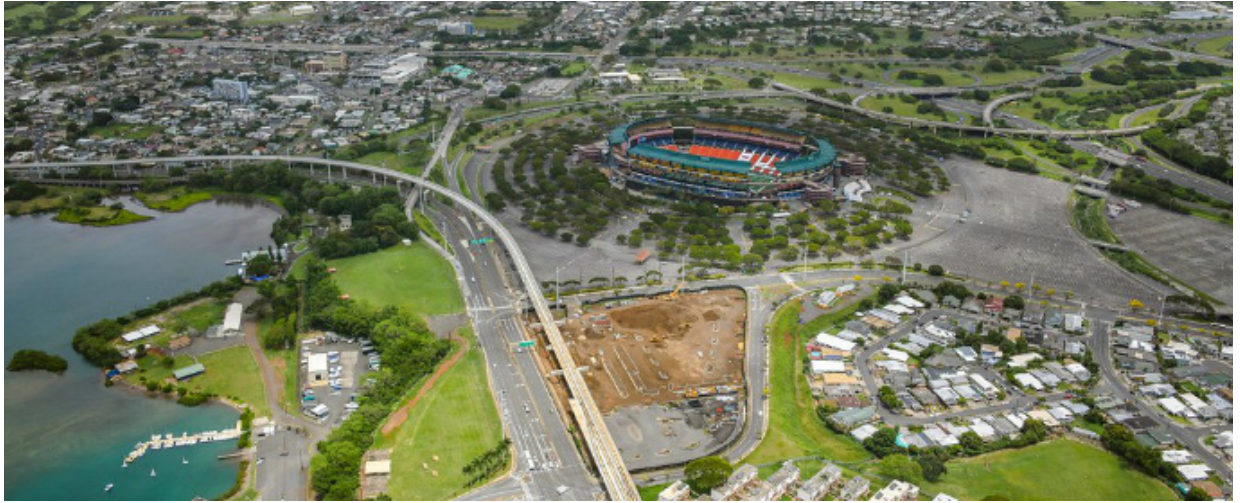
Halawa Station under construction at Aloha Stadium (HART, 2019)
