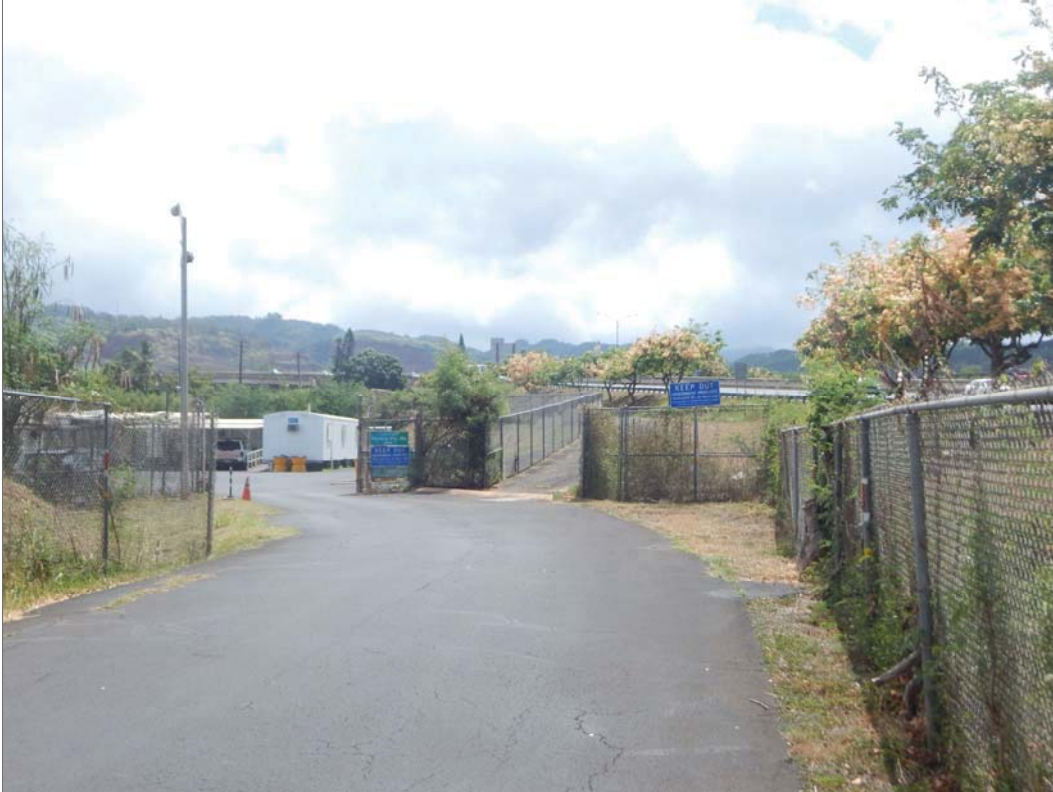
Figure 28. Entrance to HDOT field office near the confluence of the Moanalua Freeway and the H3 Freeway.
