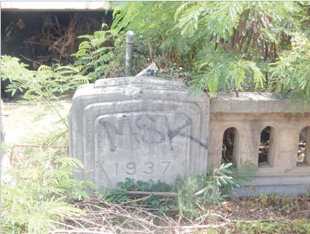
Figure 32. Date cast in Hālawā Stream bridge.
