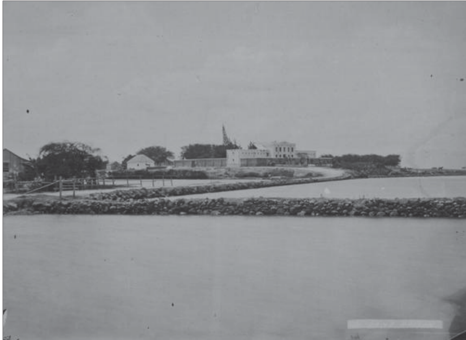
Figure 14. Former Oahu Jail in Iwilei with fishponds in foreground, Hawai'i State Archives, Oahu Prison Collection, PP-61-5-020-00001.
