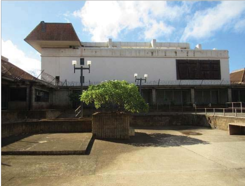
Figure 42. Current OCCC-10, original Holding Unit built ca. 1912.
