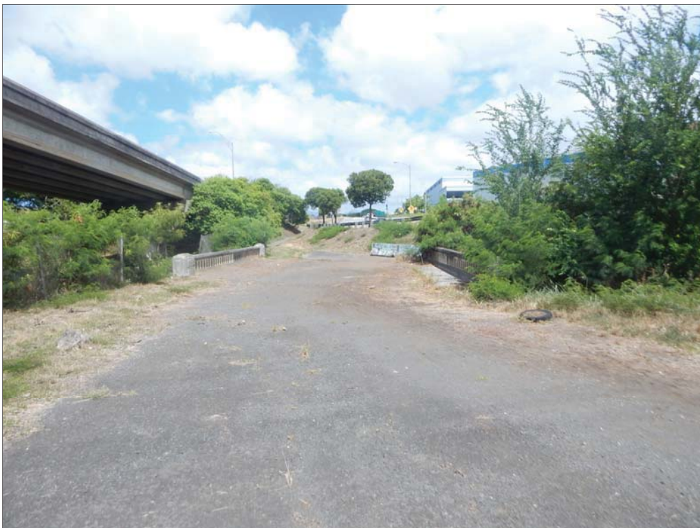
Figure 31. Bridge crossing north branch of Hālawā Stream.
