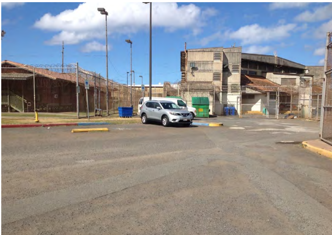
Photograph 2: Paved parking lot and facility buildings west of parking lot, view facing west
