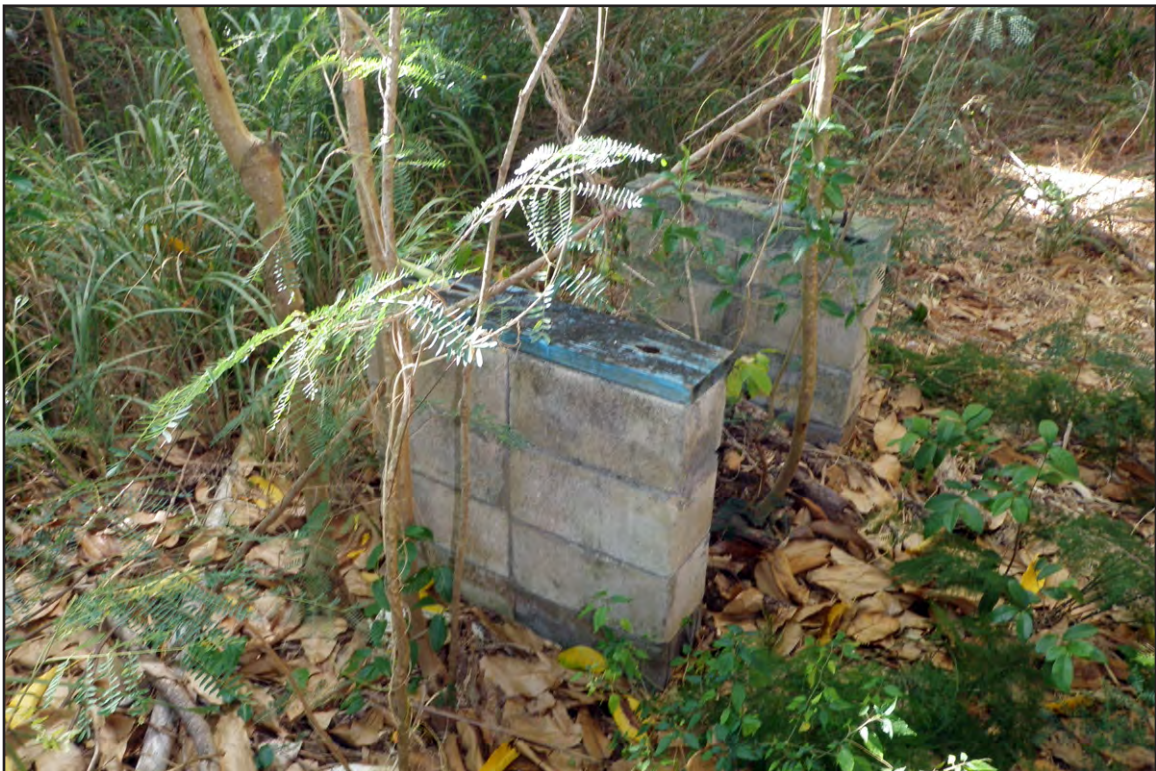
Plate 27: Concrete Block Feature at WCCC
