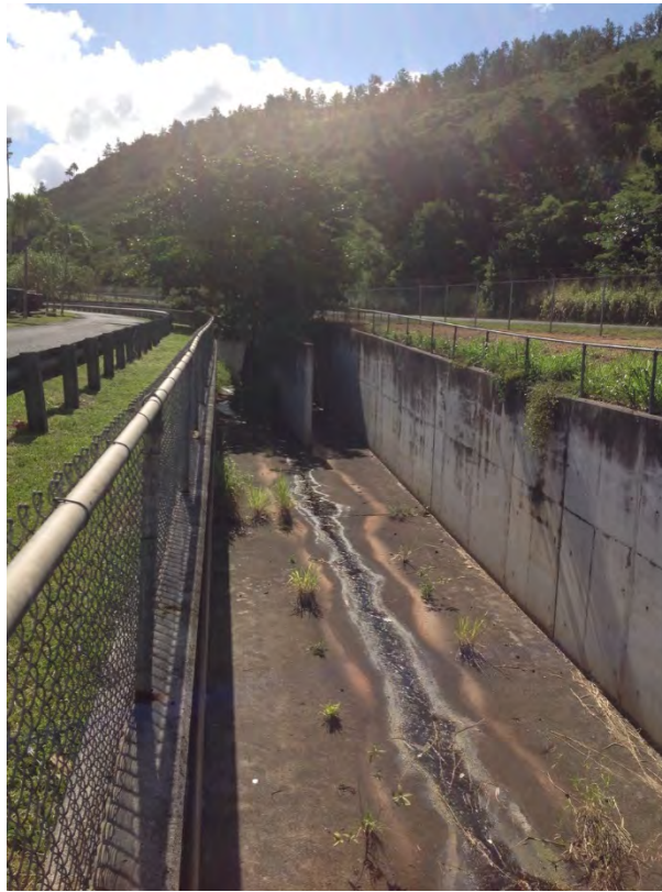
Photograph 7: Concrete-lined channel along southern site boundary
