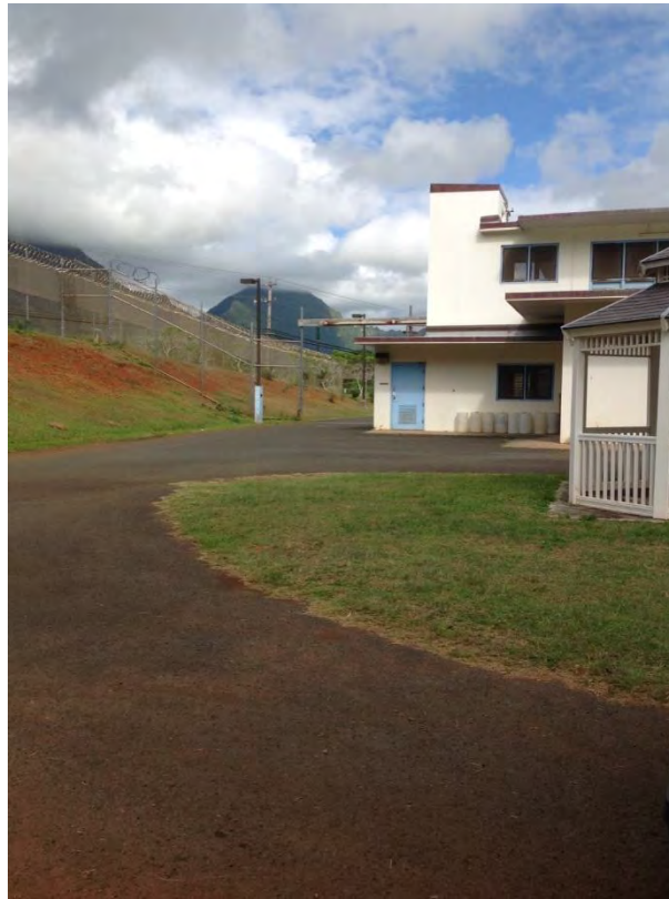
Photograph 1: View of paved parking lot and facility buildings
