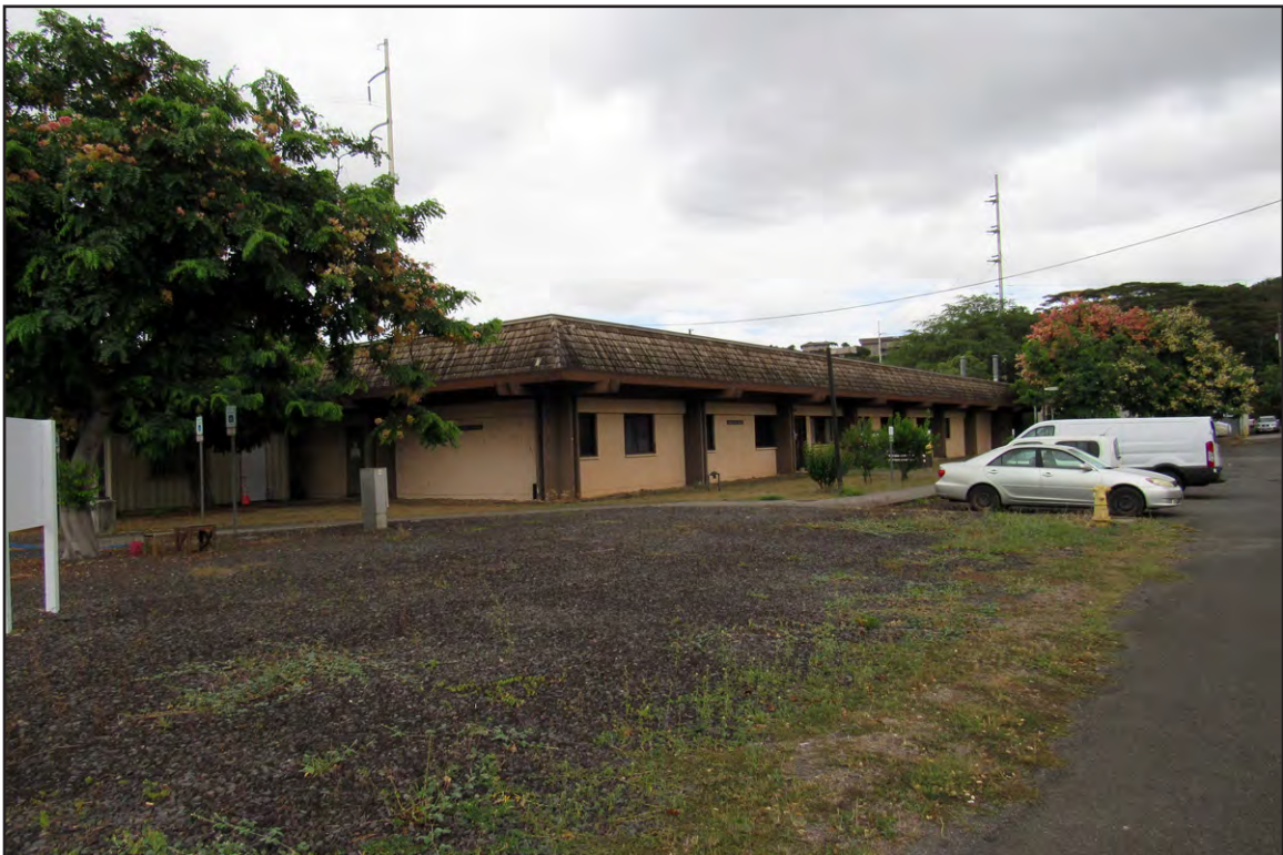
Plate 35: Laboratory Office Building, Animal Quarantine Station
