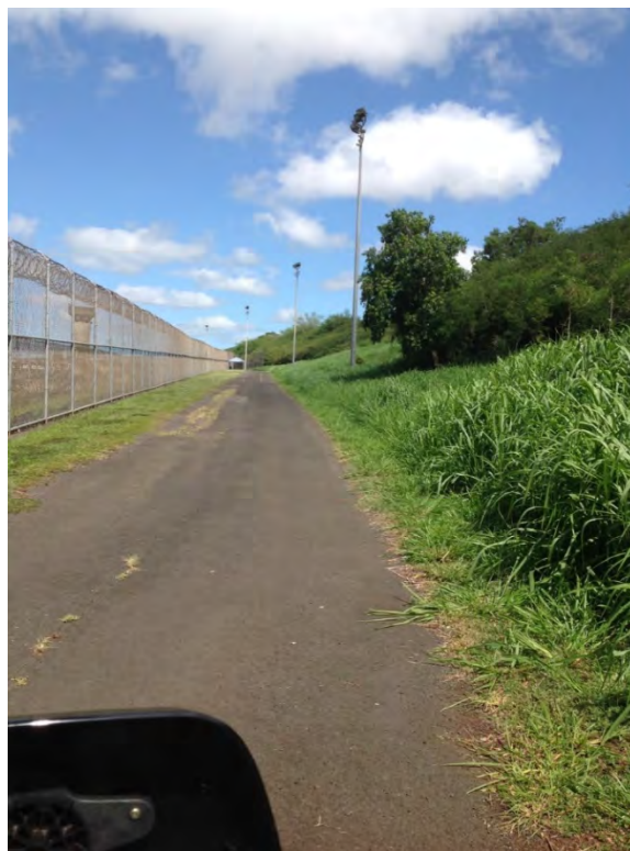
Photograph 14: View looking west along northeast perimeter road
