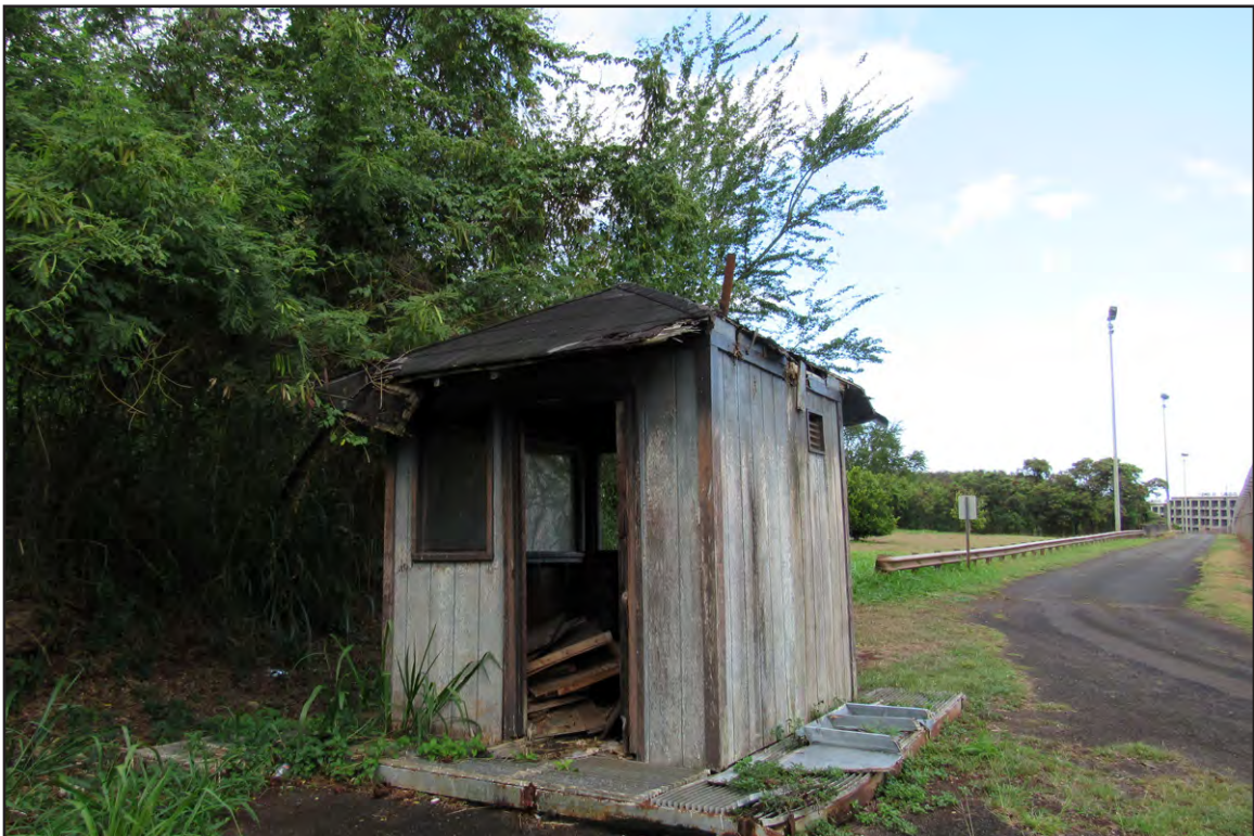
Plate 42: Abandoned Maintenance Shed, Halawa
