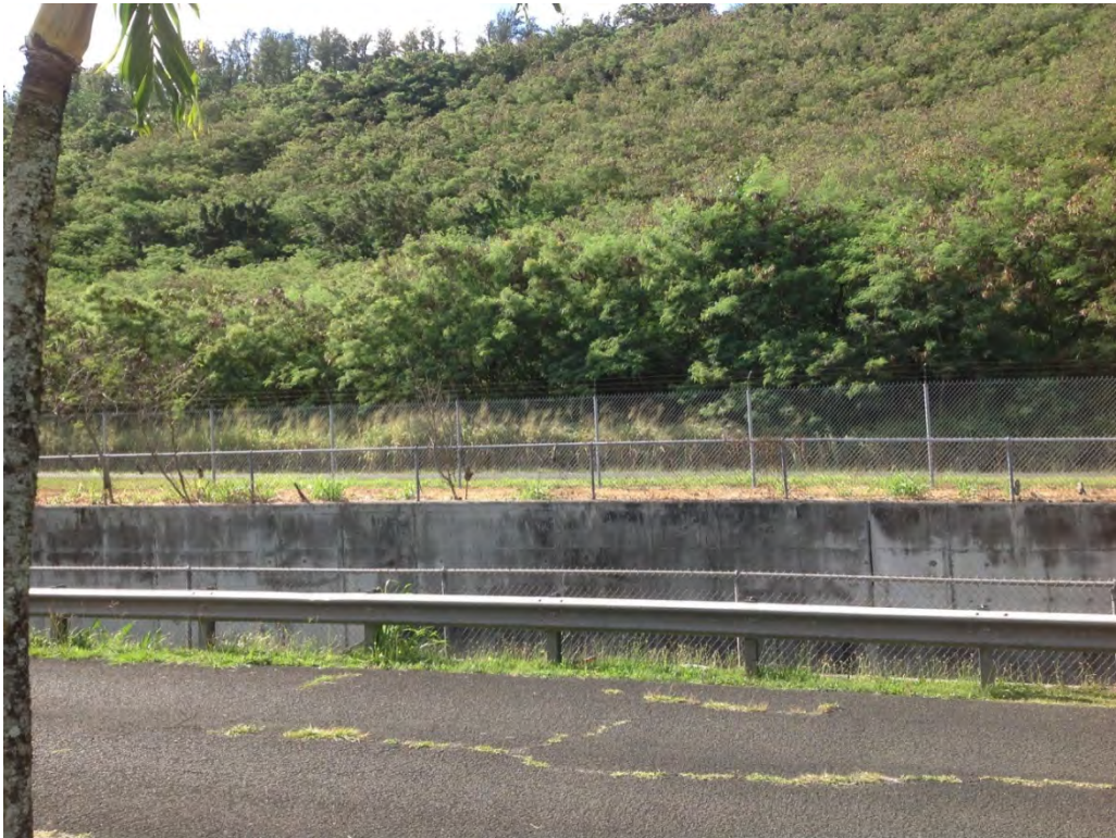
Photograph 3: View looking southeast at southern property boundary showing concrete lined channel and steep slope of adjacent property
