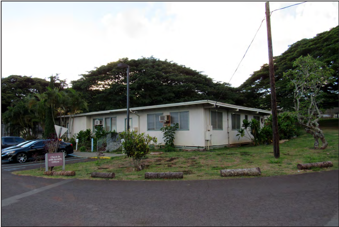
Plate 62: Administrative Building, WCCC
