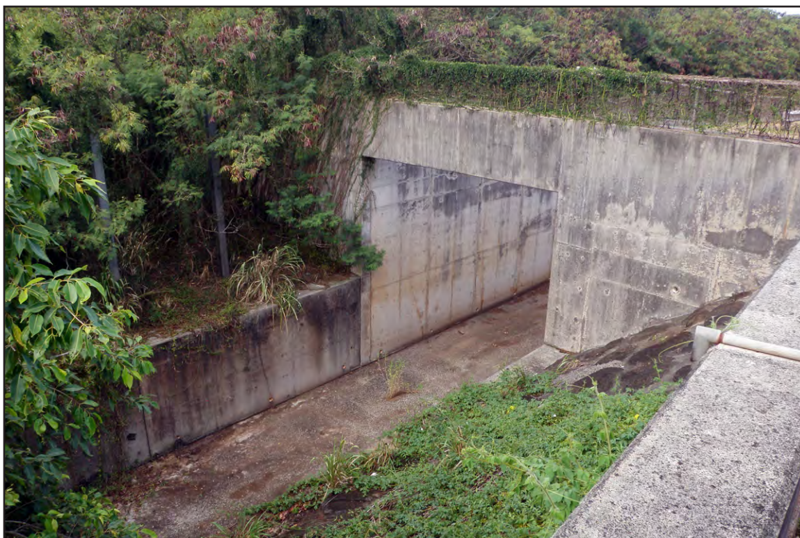
Plate 13: Concrete Drainage Flue Along Southern Perimeter of Halawa Correctional Facility
