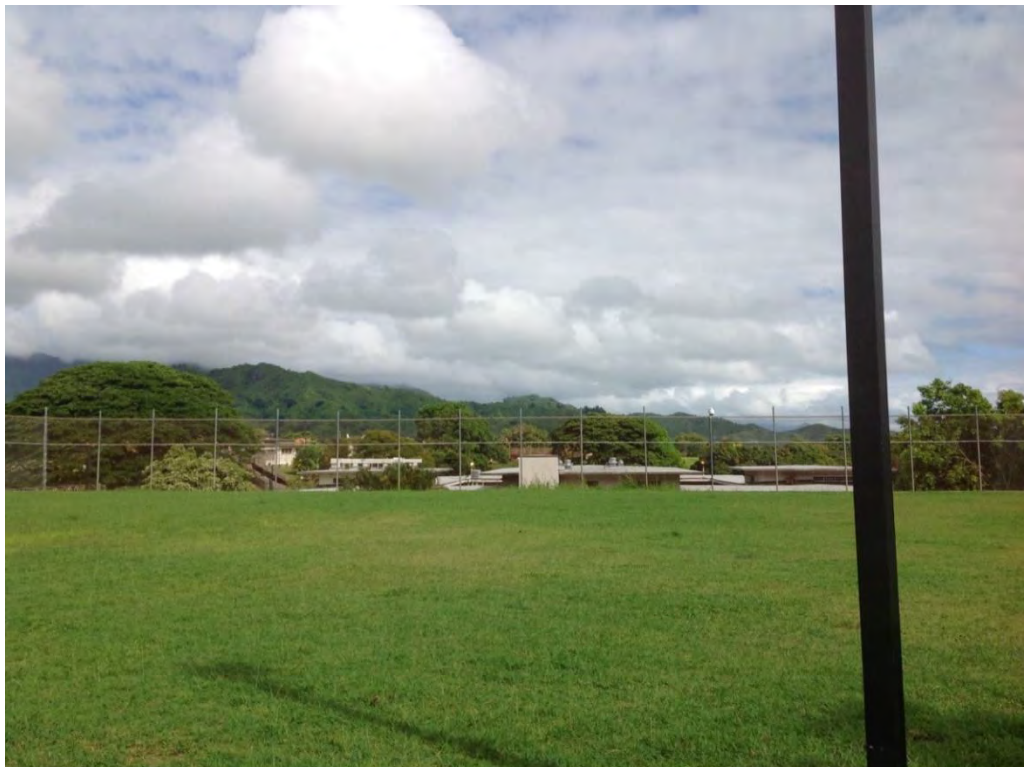
Photograph 2: Recreational field with facility buildings in background, view facing northeast
