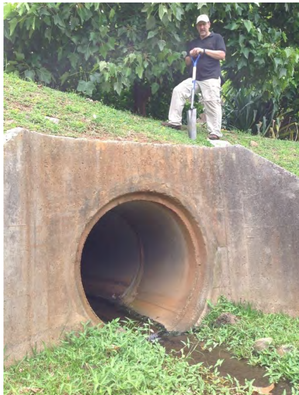
Photograph 14: Culvert at southern end of stream
