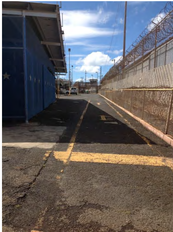
Photograph 7: Paved access road along southwest perimeter
