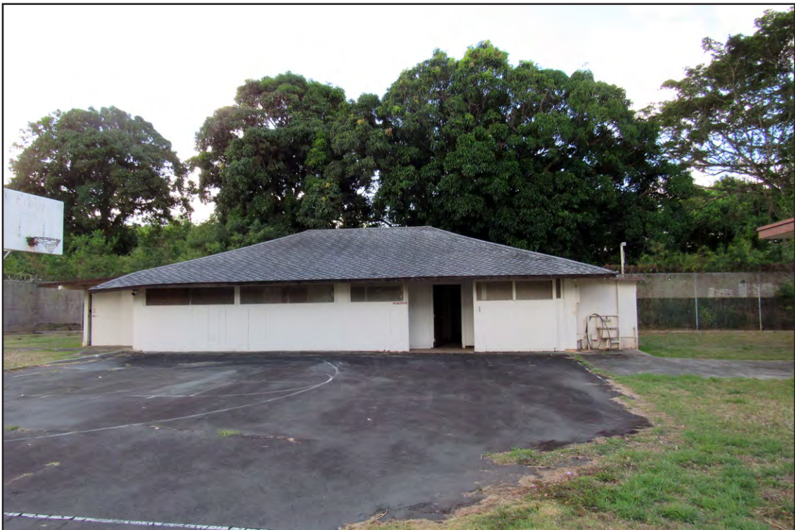
Plate 63: Hookipa Cottage Auxiliary Building, WCCC
