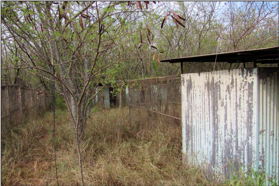
Plate 6: Field Conditions at Animal Quarantine Station North of Administration Building
