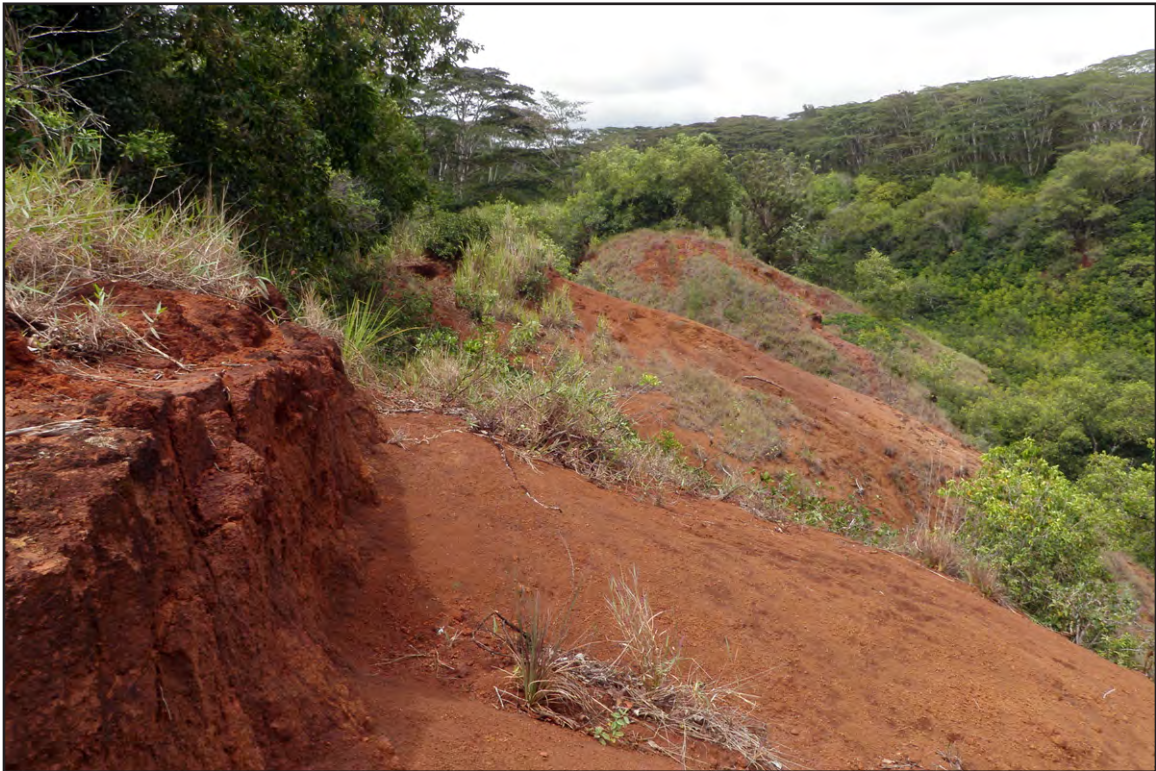
Plate 19: View of Exposed Southeast Edge of Landform at Mililani Technology Park Lot 17
