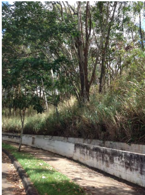
Photograph 14: View looking west along southern property boundary adjacent to Wikao Street
