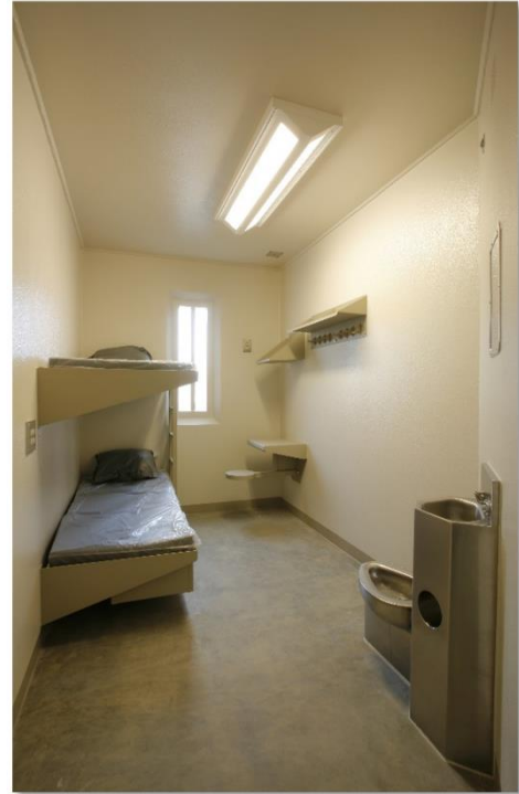
TYPICAL TWO-PERSON CELL WITH BUNKS, WRITING SURFACE, PLUMBING FIXTURE, GROOMING AND UNENCUMBERED SPACE
