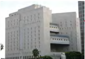
Los Angeles Metropolitan Detention Center
