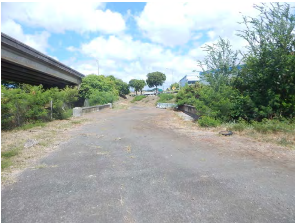
Figure 31. Bridge crossing north branch of Hālawā Stream.
