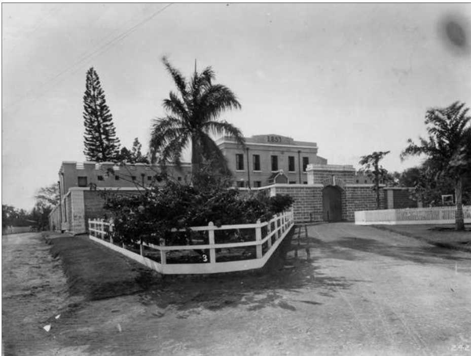
Figure 15. Exterior of former Oahu Prison, Hawai'i State Archives, Oahu Prison Collection, PP-61-5-005-00001.
