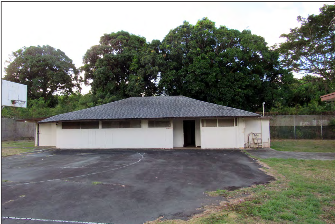
Plate 63: Hookipa Cottage Auxiliary Building, WCCC
