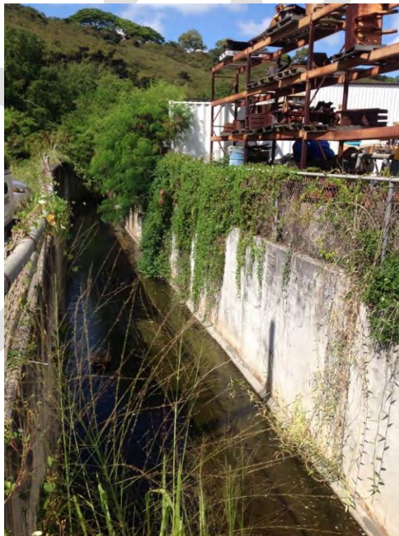
Photograph 6: Concrete-lined channel along western boundary, view looking south
