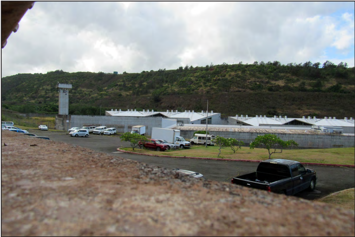
Plate 39: Medium Security Facility, Near Administration, Halawa
