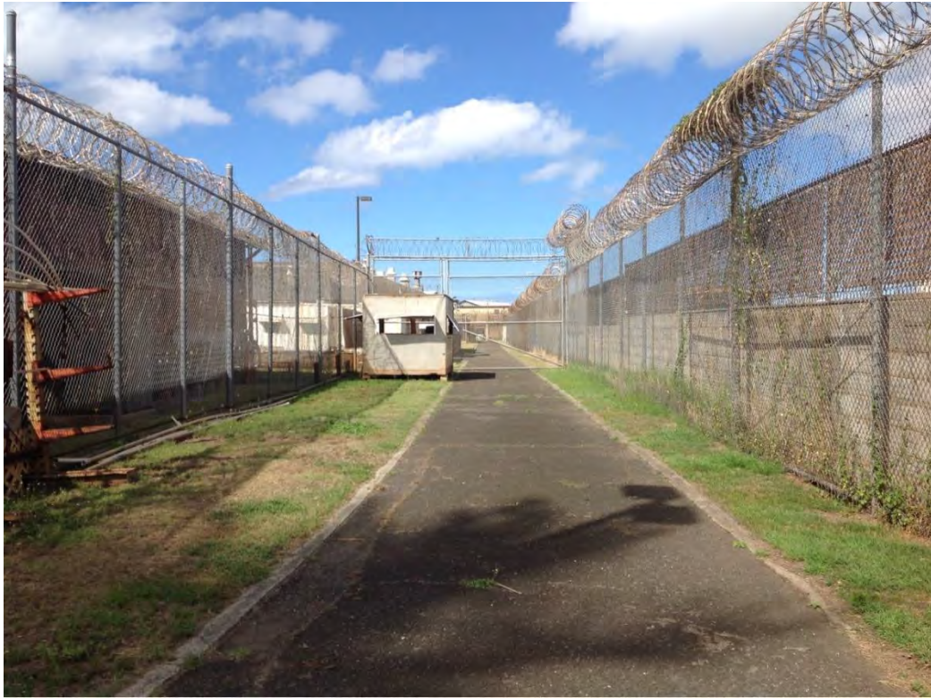
Photograph 3: View from northwest corner, facing southwest along perimeter road
