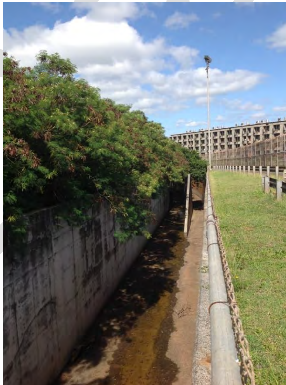
Photograph 8: Concrete-lined channel along east boundary, view looking southwest
