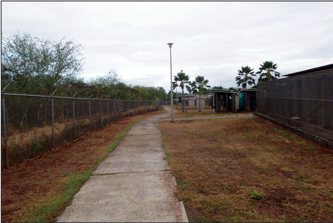
Plate 5: Field Conditions at Animal Quarantine Station South of Administration Building
