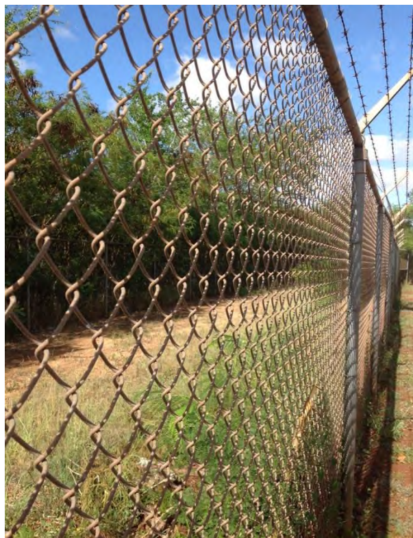
Photograph 2: Fire break along southern site boundary, view facing west
