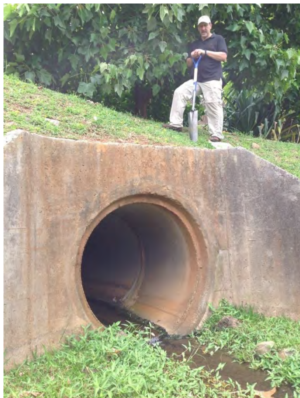
Photograph 14: Culvert at southern end of stream
