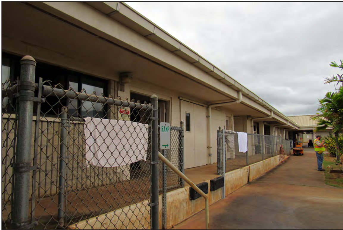
Plate 32: Public Service Desk Building, Animal Quarantine Station, Facing East
