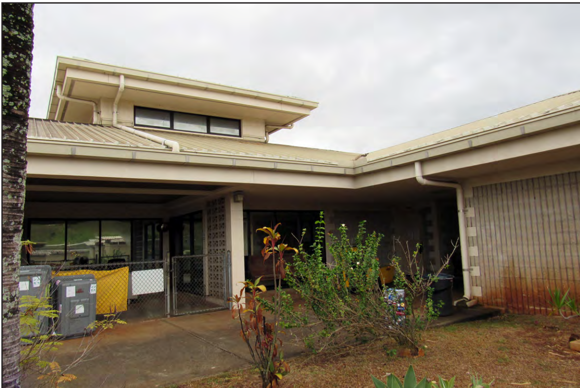
Plate 31: Public Service Desk Building, Animal Quarantine Station, Facing North
