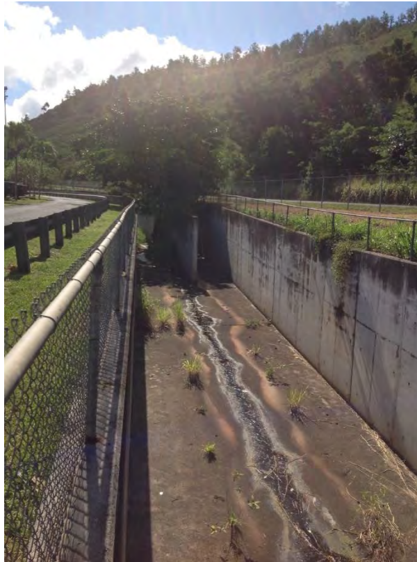
Photograph 7: Concrete-lined channel along southern site boundary
