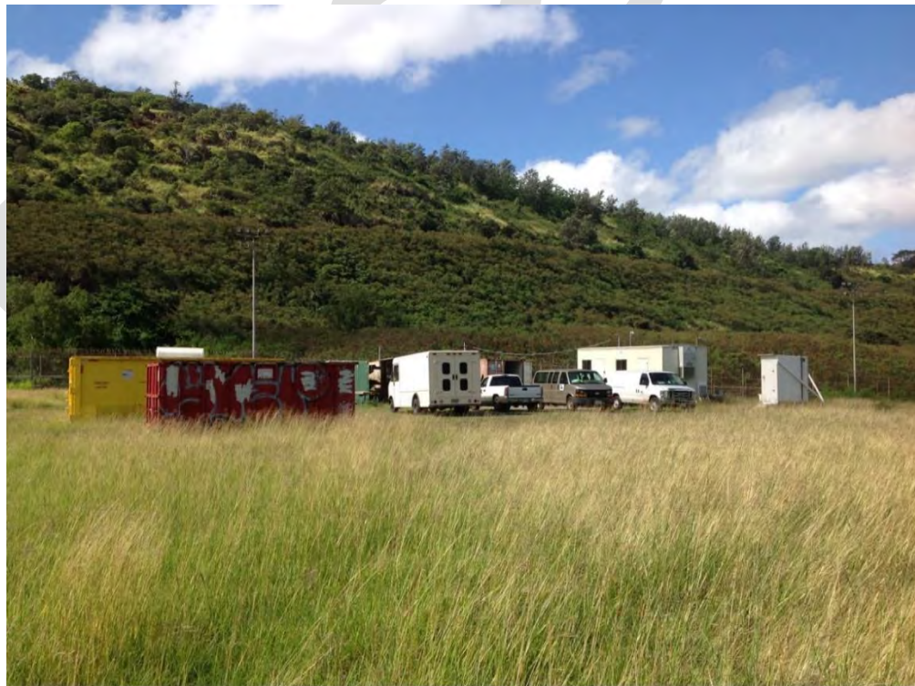
Photograph 4: View of recreational field with construction staging/storage area
