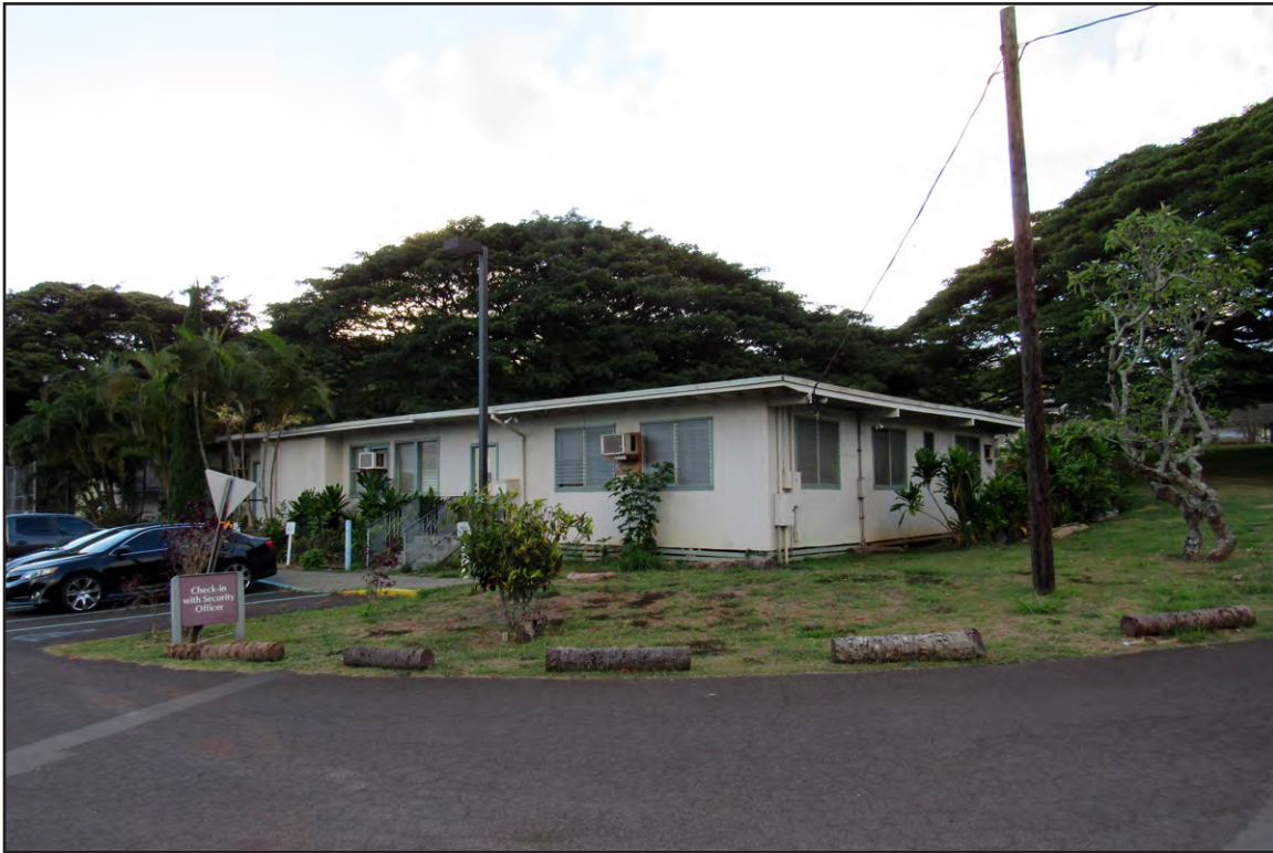
Plate 62: Administrative Building, WCCC
