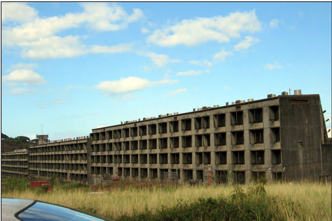
Plate 40: Medium Security Facility Cell Block, Halawa
