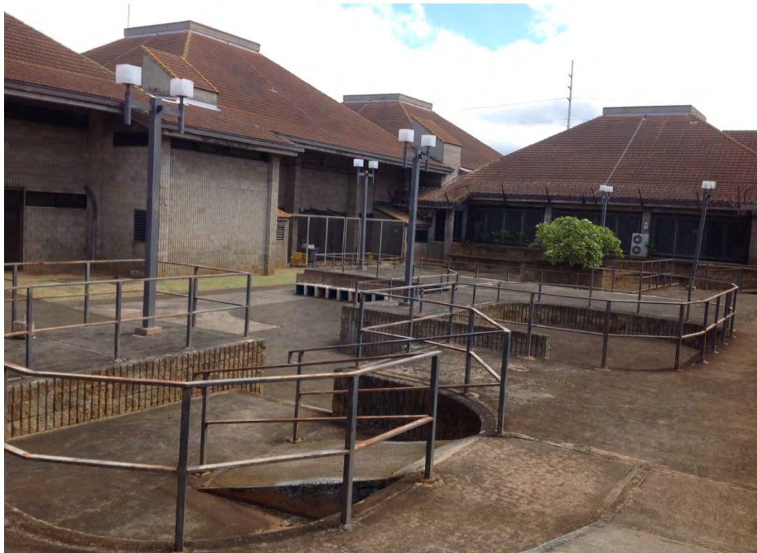
Photograph 10: Outdoor visiting area in center of facility
