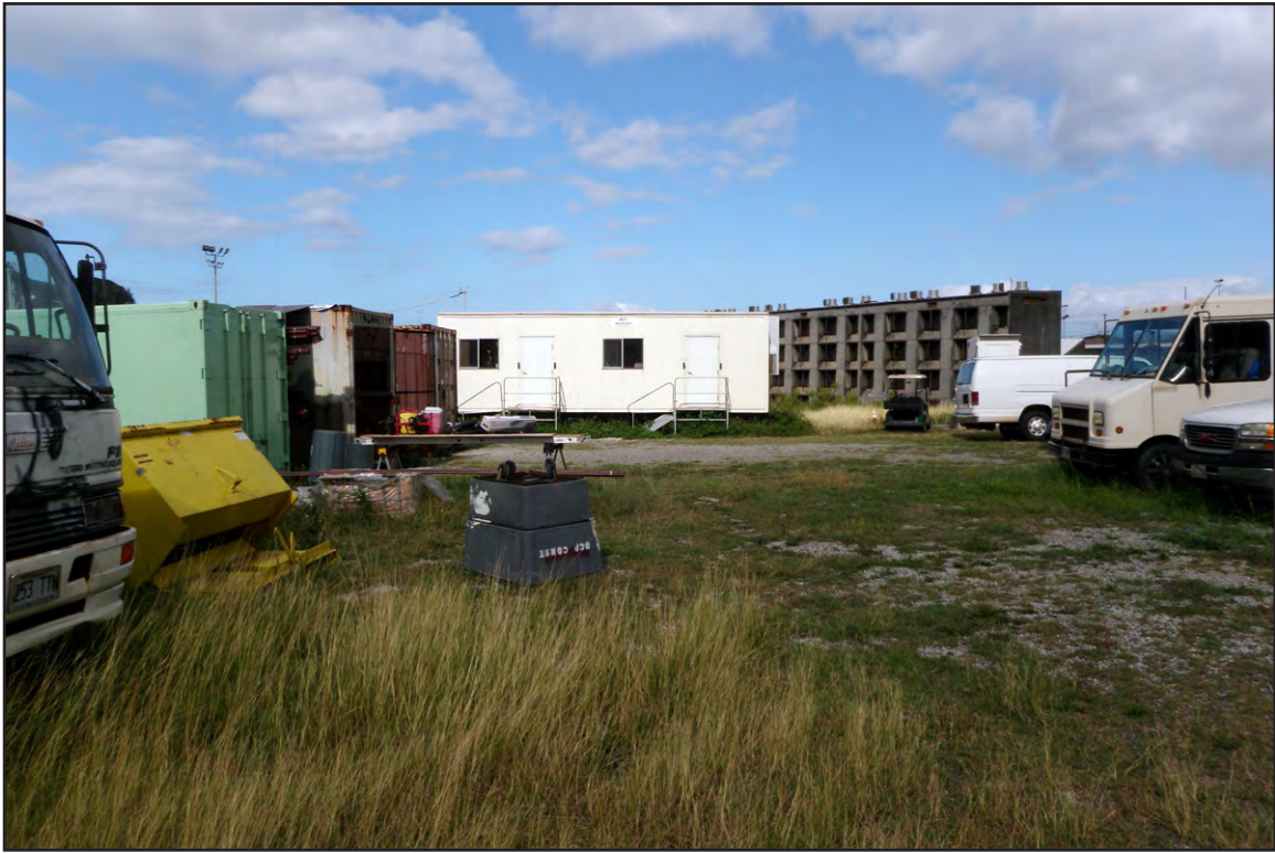
Plate 11: Temporary Structures and Graveled Surface at West End of Recreation Yard, Halawa Correctional Facility
