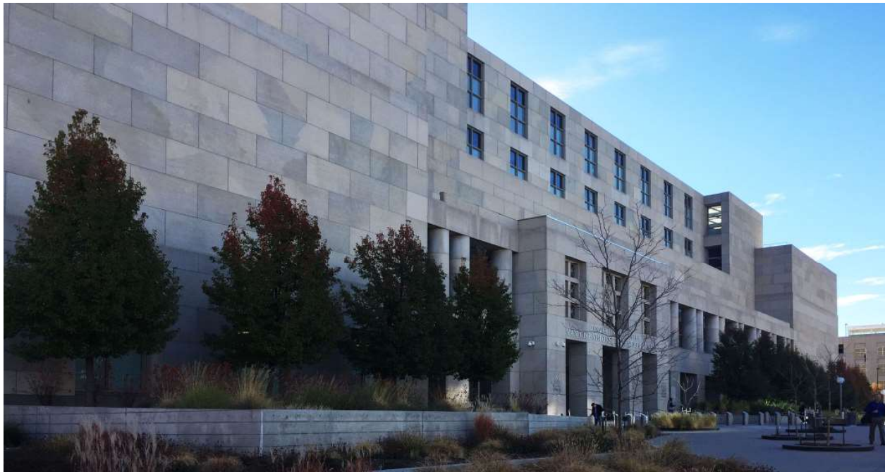
Van Cise-Simonet Detention Center
