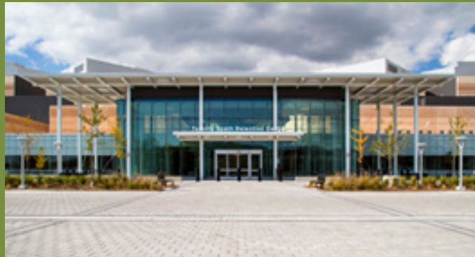
Toronto South Detention Centre, Canada
