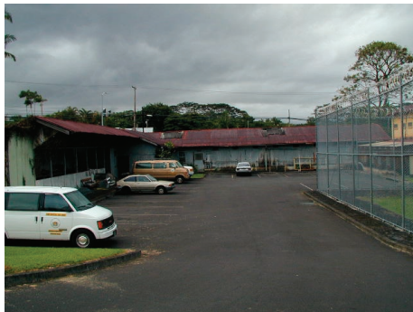
Hawaii Community Correctional Center
