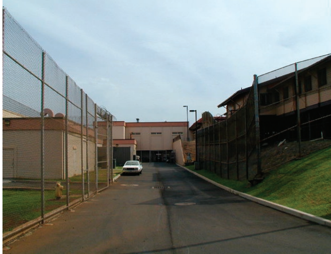
Exterior view of Maui Community Correctional Center
