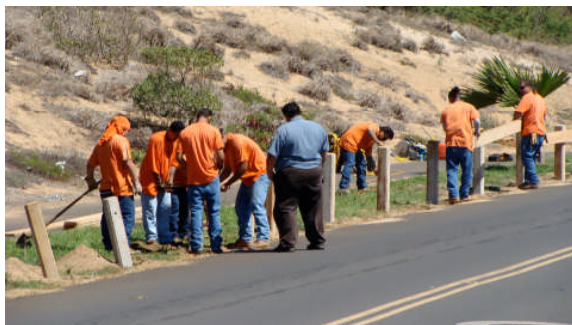
MCCC workline inmates installed posts and rails along Keopulani Park Drive.
